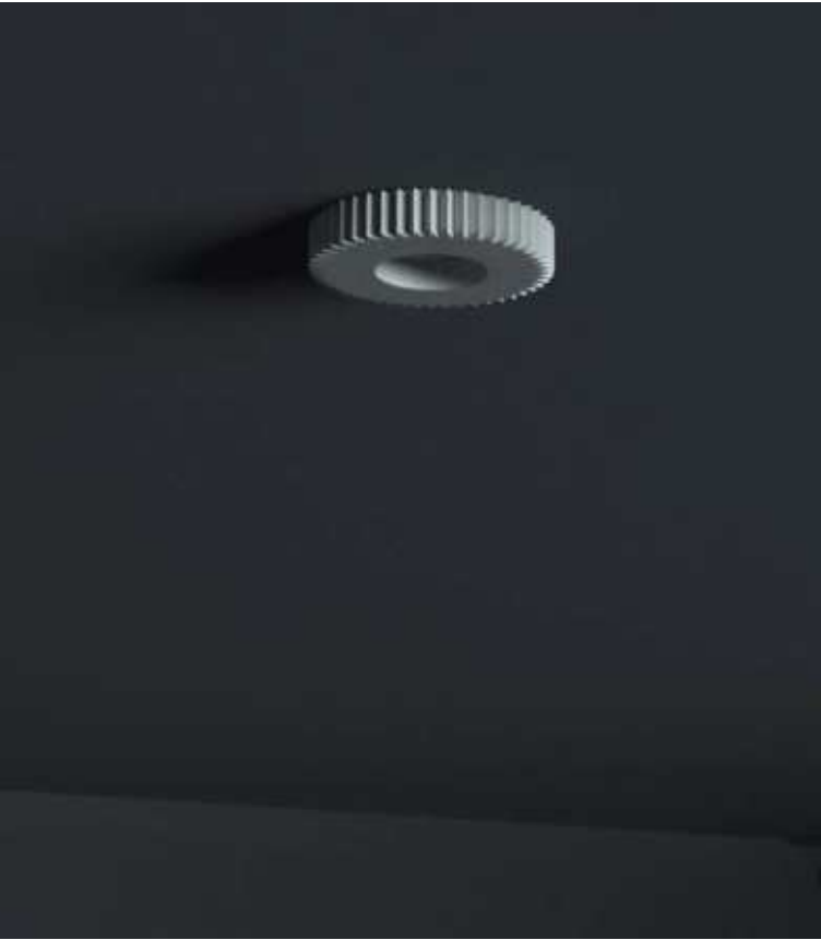
Base of the overflow drain
